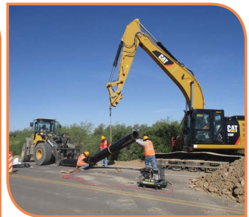
Avondale 127 th Avenue Waterline Improvements
